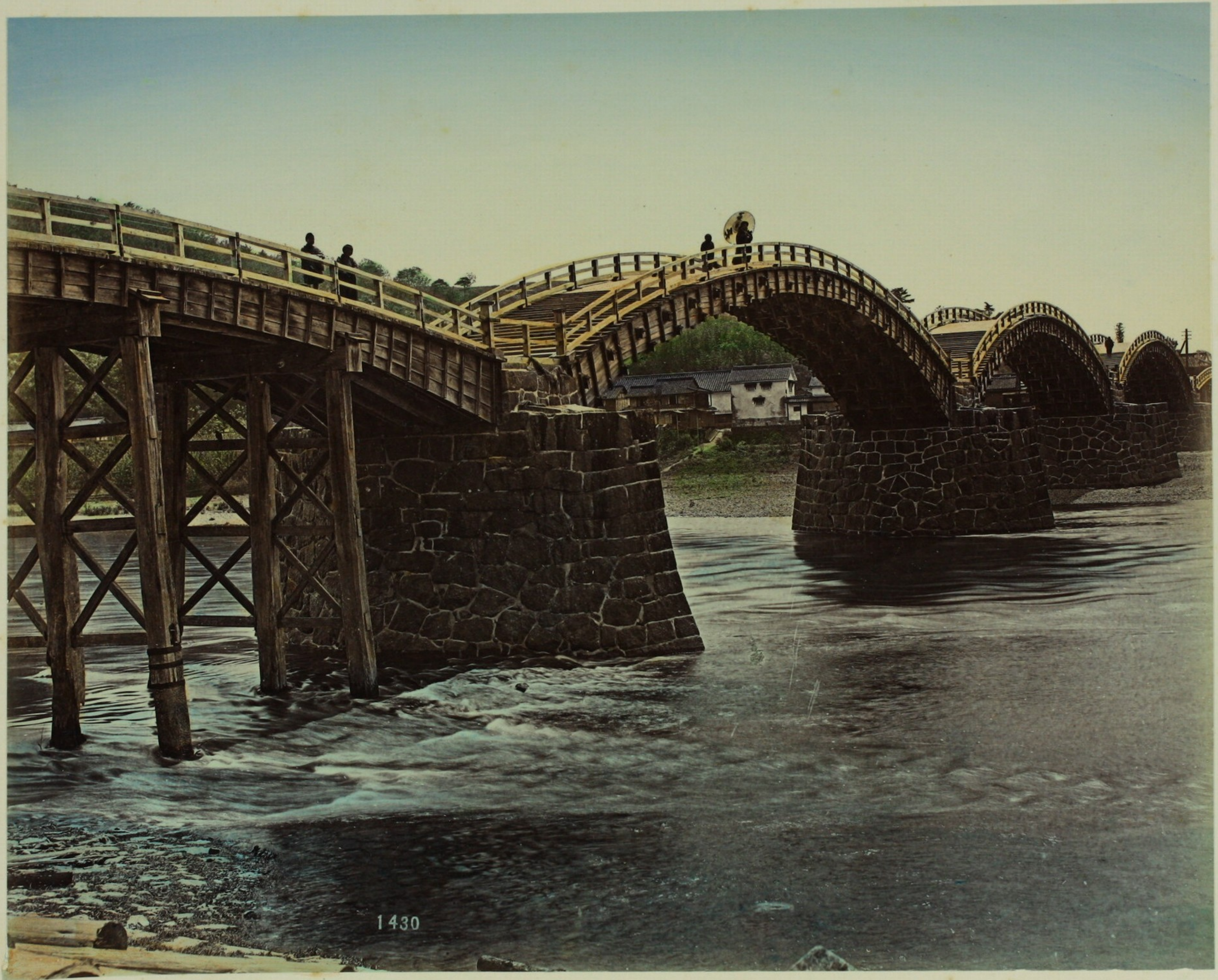
VIEW OF KINTAI BASHI BRIDGE AT IWAKUNI.
