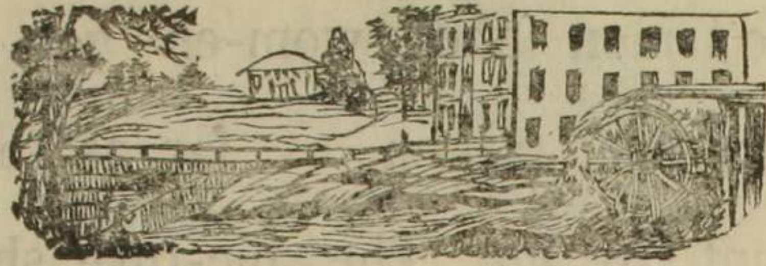
The Mill-stream and Flour-Mill.
