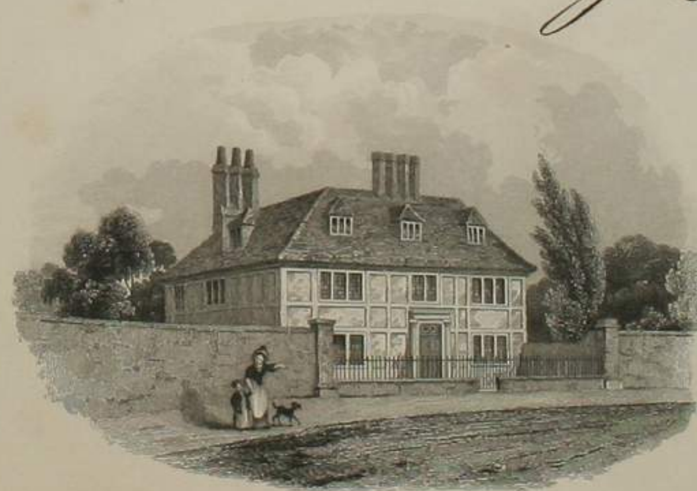
THE RESIDENCE OF JOHN HOWARD AT CARDINGTON, BEDFORDSHIRE.
